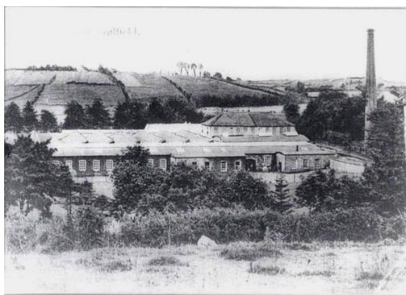
Acheson and Smith Weaving Plant, Castlecaulfield
